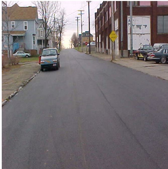
Seneca Ave. after paving.
